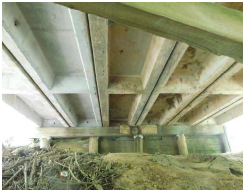
BOTTOM DECK SPAN 1
