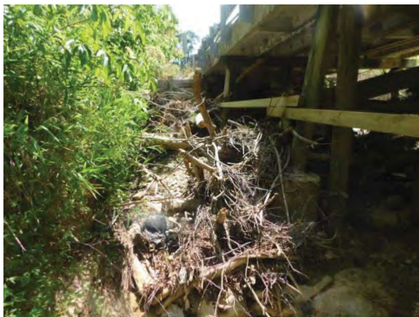
LEFT SIDE DRIFT INLET END
