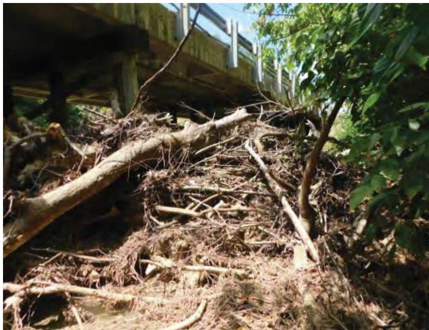
LEFT SIDE DRIFT INLET END
