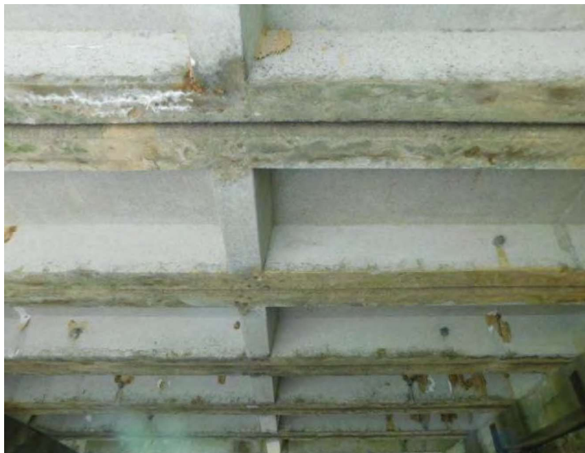
BOTTOM DECK SPAN 4
