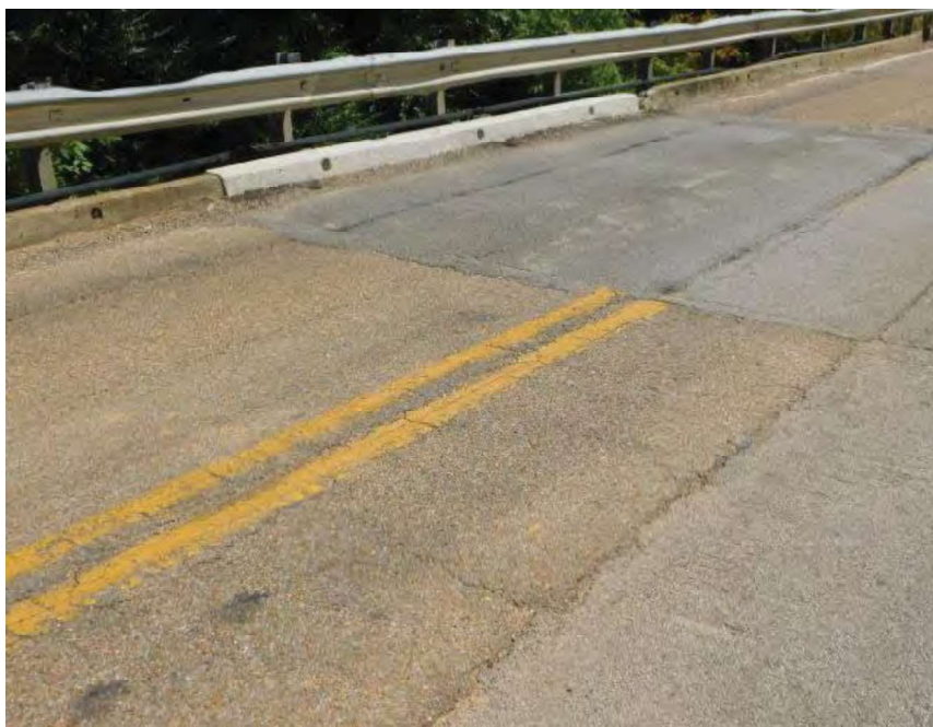
VIEW ACROSS TOP OF DECK
