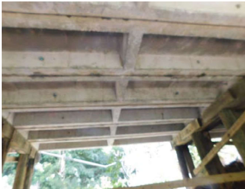
BOTTOM DECK SPAN 2
